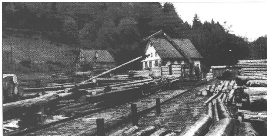
Log handling carriage in the Roth family sawmill at Schapbach
