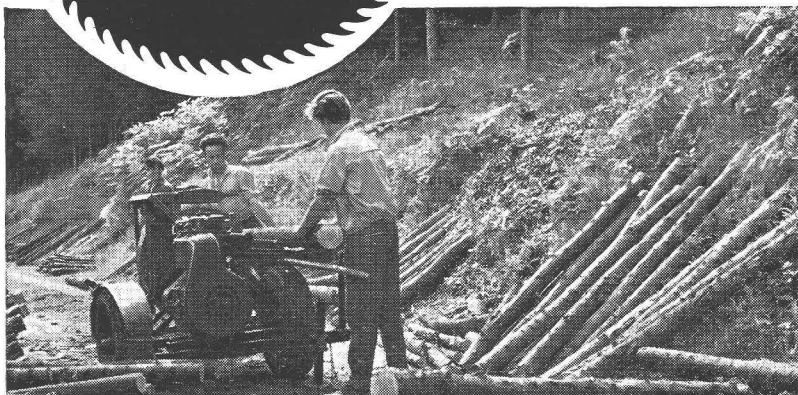
One of a fleet of McConnell Mobile Saws employed by Powell Duffryn Timber Industries Ltd. for cutting pit props in the Welsh forests. (Photo by courtesy of Powell Duffryn Ltd.)
