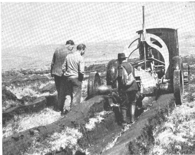
"THE MACHINE AND ITS JOB."
