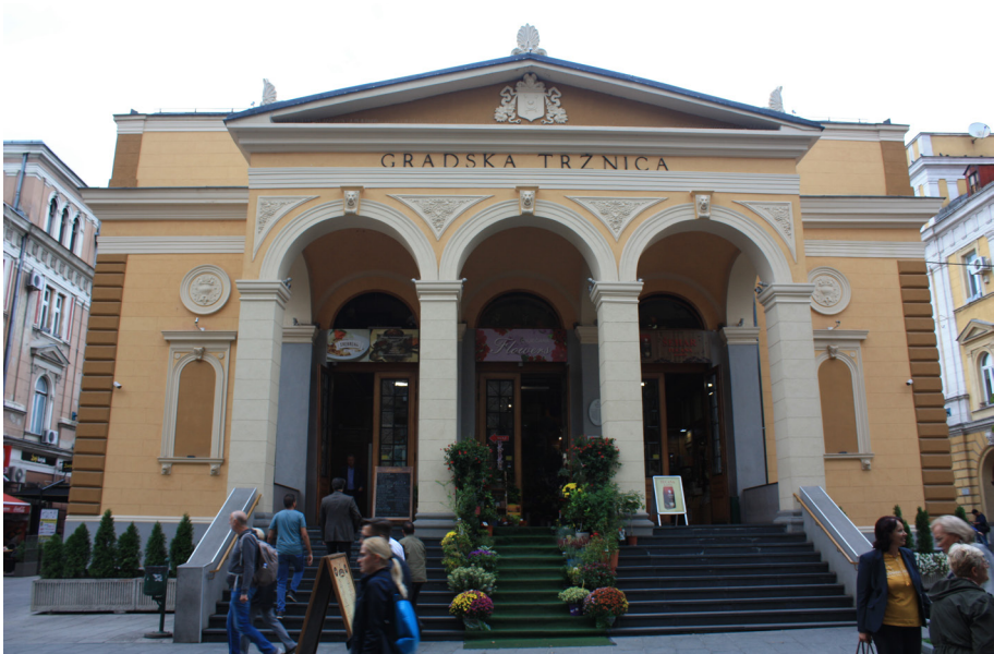
Figure 7: The rebuilt Markale Market House which is now a national monument.
