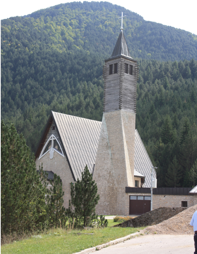
Figure 1: The wooden steeple of St. Elijah's Church at the Franciscan monastery complex in Blidinje Nature Park. This wooden structure was designed to enhance the musical tone of the church bells.
