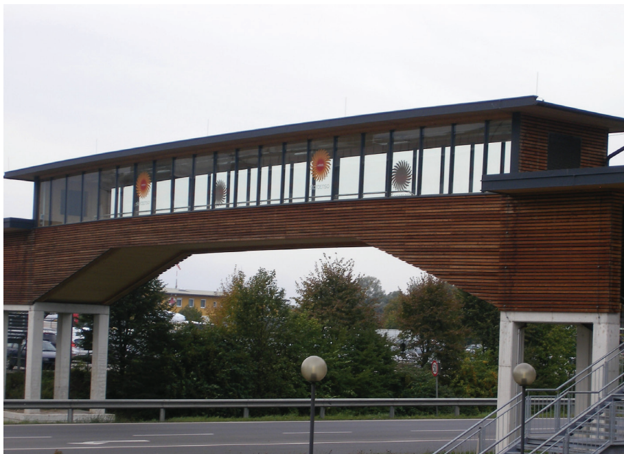
Figure 6: Demonstrating confidence in their product! Note the absence of any intermediate support structure on a CLT footbridge which spans a four-lane highway beside the Stora Enso sawmill at Ybbs an der Donau.
